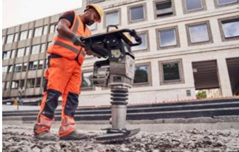
Especially on inner-city construction sites, the battery-powered rammers emit less noise and emissions and thus protect the construction site environment.
