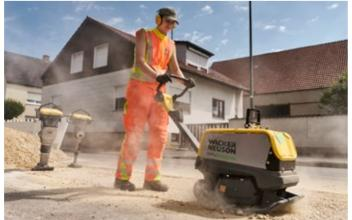
With one battery charge, the APU3050e compacts up to 333 m<sup>2</sup> soil\*.
